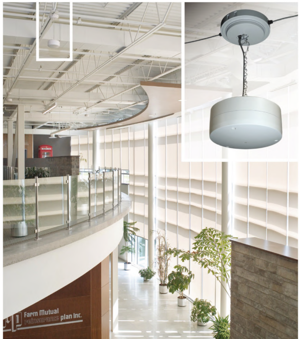
Photo courtesy of K.R. Moeller Associates Ltd.
