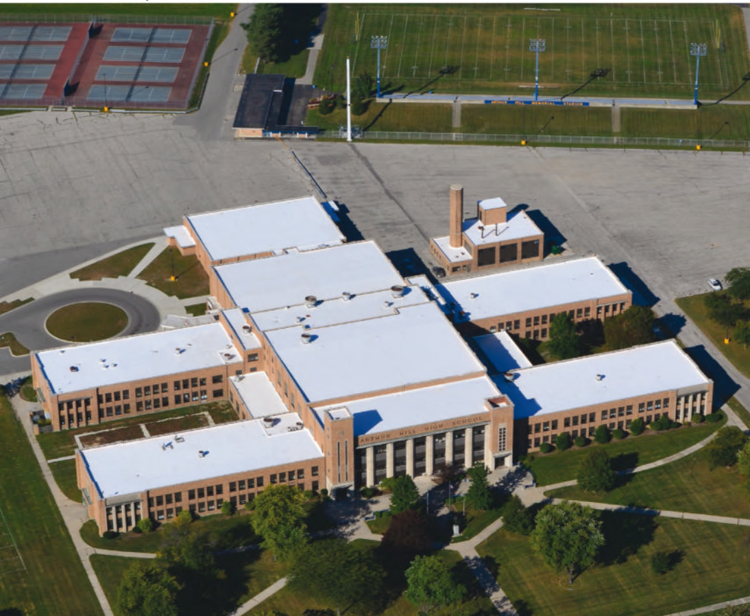
Cool roofs deflect solar energy away from a building and back to the atmosphere and beyond.
