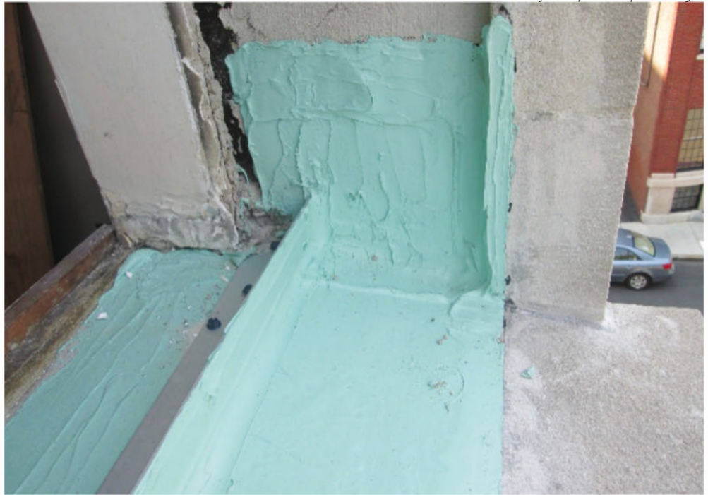
Liquid flashing installation at window opening—single material and installation operation.
