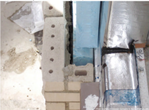
Self-adhered membrane installation at window opening—multiple layers and sequencing implications.
