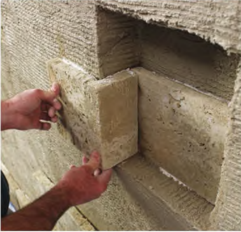
Wall transition using manufactured stone corner pieces.
